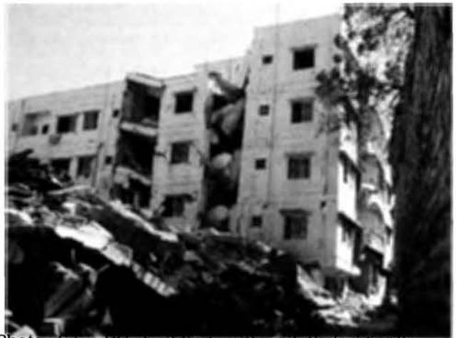
Photo 6.5. RC building with piloti (originally classified as Class C, but in reality weaker than Class C)
