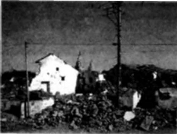
Photo 6.8. Damage of masonry dwellings in Loria,  $Q_{MSK2}=8.9$ .
