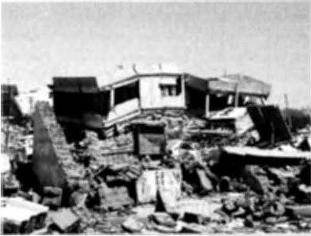
Photo 6.6. Damage to a RC building in Bhachau
