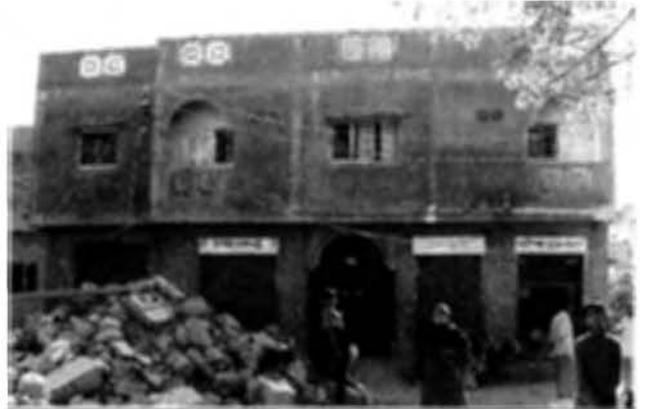
Photo 6.4. RC building without piloti (Class C)
