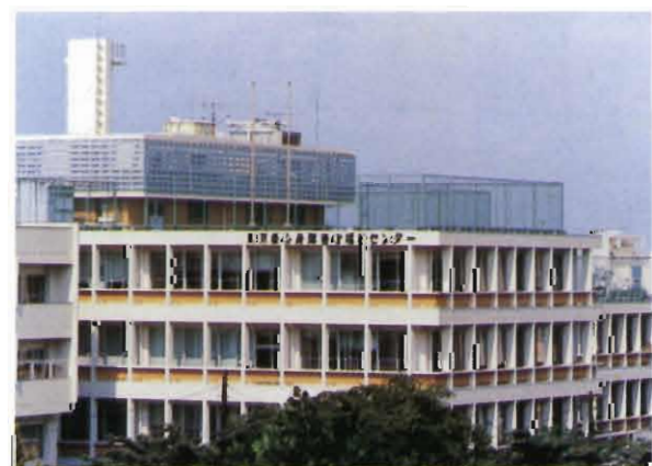
23. Tokyo Metropolitan Rehabilitation Center for the Physically and Mentally Disabled – building
