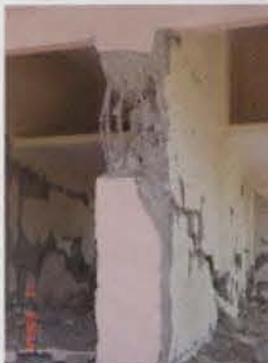
Photo 7.9. Shear failure of columns in Pooja Flat (page 80).
