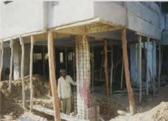
Photo 7.42. Repair work under progress of the damaged columns of the open-first-story of a 4-story apartment building in Ahmedabad (page 103).
