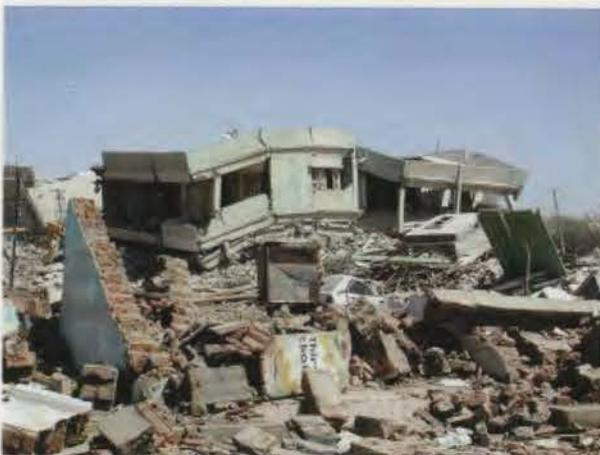
Photo 6.6. Damage to a RC building in Bhachau (page 63).
