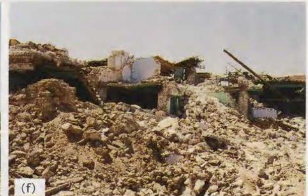
Photo 7.30. Towns where a large number of masonry houses collapsed (page 94).
