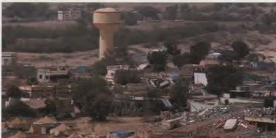
Photo 8.15. Non-damaged typical elevated water tank in Bhachau (page 114).
