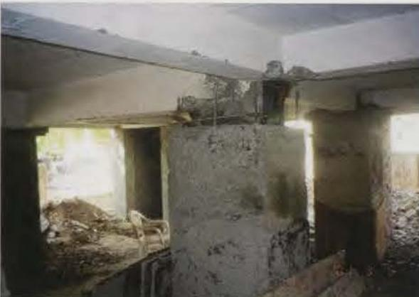
Photo 7.44. The connection between the reinforcement of the column of first story and the floor-beam of the second story was inadequate, leading to weak beam-column joint (page 104).
