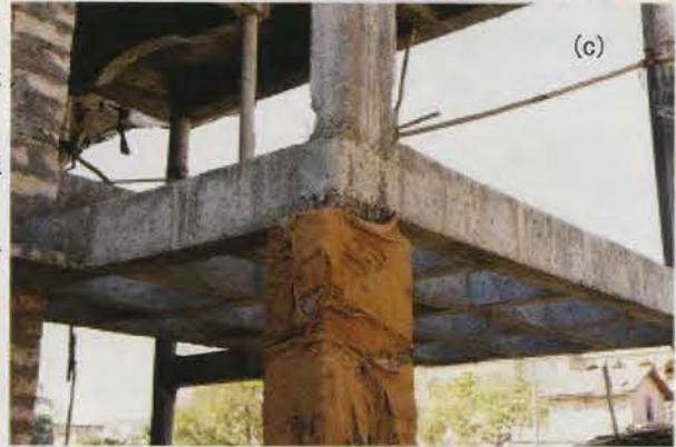
(c) Close up of the RC column (It is very slender and joint connection is poorly constructed.)
