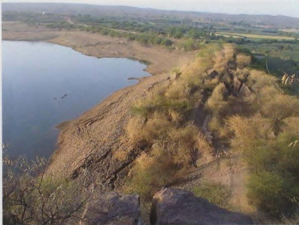
Photo 4.4. Bird's eye view of a large surface crack with a length of about 350 m, whose left portion slid down partially to the lake-side (page 50).
