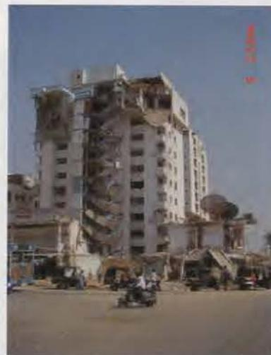
Photo 7.5. Mansi Complex collapsed because of the too much load from the pool at the top (page 78).
