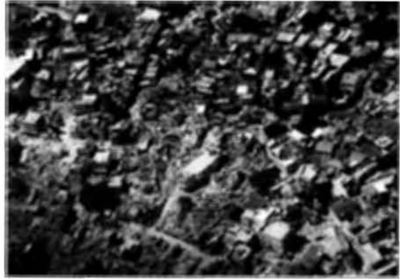
Photo 2.19. Aerial view of damage at Anjar. Note that only the centre of the town was seriously affected by this quake.
