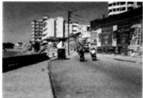
Photo 2.21. Alampana Fort after the earthquake.
