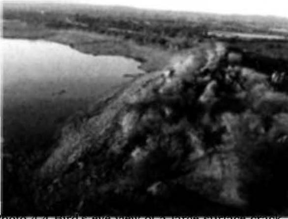
Photo 4.4 Bird's eye view of a large surface crack with a length of about 350 m, whose left portion slid down partially to the lake-side.
