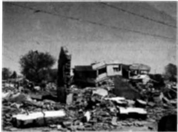
Photo 5.2. Collapse of RC and masonry buildings in Bhachau center.
