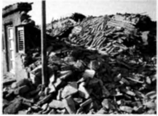
Photo 4.2 Completely destroyed houses with stone masonry and mud mortar.
