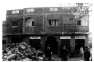
Photo 6.4. RC building without piloti (Class C)
