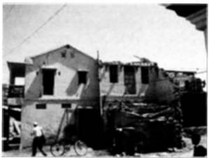
Photo 6.11. Damage of masonry building in Mundra, Q\_MSK2=7.6.
