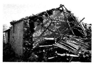
Photo 6.1. Type 1 masonry house (Class A)
