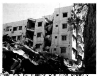
Photo 6.5. RC building with piloti (originally classified as Class C, but in reality weaker than Class C)
