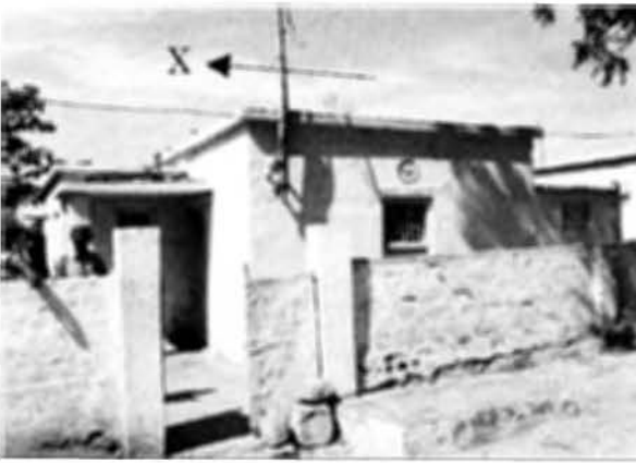
Photo 7.36 Microtremor measurements at a single-story masonry building
