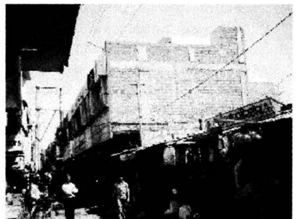
Photo 7.14. Buildings along the center street in the old town of Gandhidham (side view)
