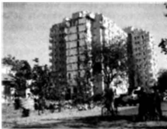
Photo 7. 2. Typical eleven-story RC building.
