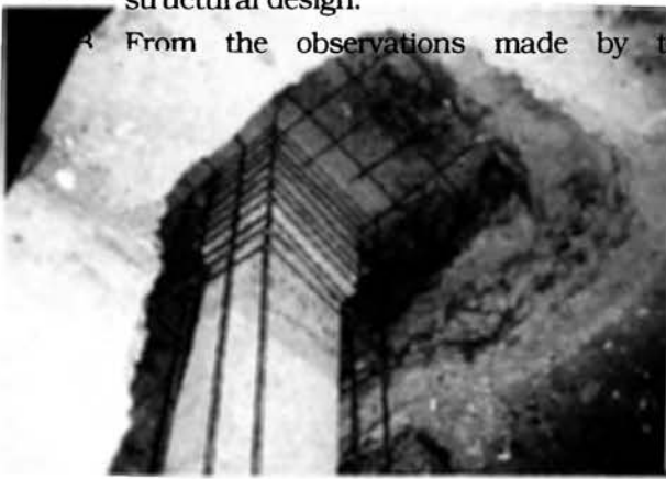
Photo 7.43 Reinforcement was extended to the footing that would considerably increase the load bearing capacity of columns.
