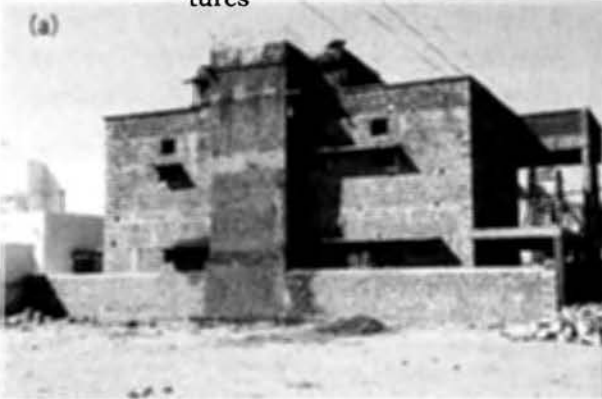
Photo 7.19 Different construction stages of largerubble stone masonry structures
