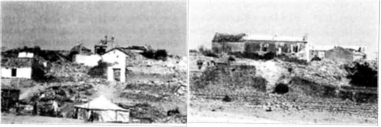
Photo 7.29 Topography induced local site effects caused extensive damage at this area located on top of a hill
