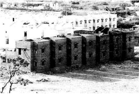
Photo 7.19 Different construction stages of largerubble stone masonry structures
