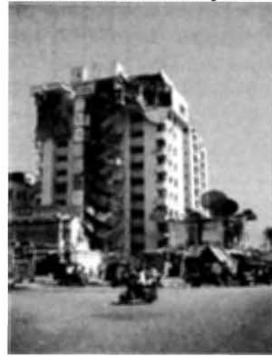
Photo 7.5. Mansi Complex collapsed because of the too much load from the pool at the top.
