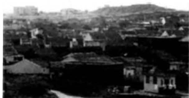
Photo 7.17 Overview of the typical town constituted by low rise masonry structures
