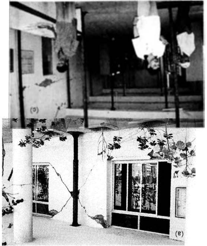
Photo 7.31 Damaged two-story RC frame houses with infill bricks (poor connection joints between column and beam, beam and wall, and column and wall)
