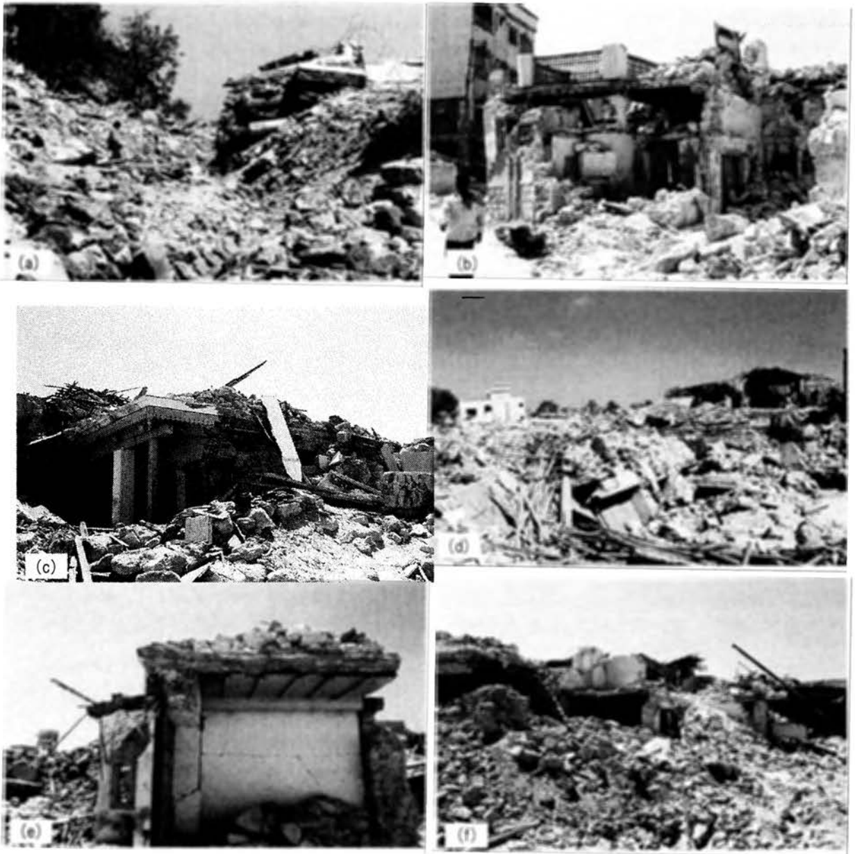
Photo 7.30 Towns where a large number of masonry houses collapsed
