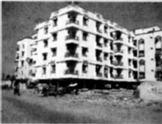
Photo 7.1. Typical five-story RC building.
