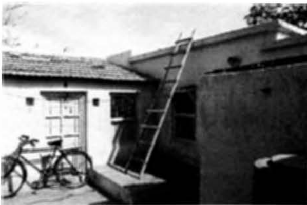
Photo 7.16 Single-story brick masonry house constructed in 1956
