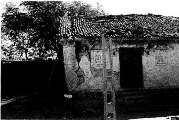
Photo 7.25 Separation of adjacent walls of a rectangular shaped dwelling
