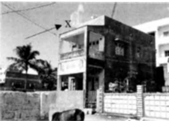
Photo 7.37 Microtremor measurements at a two-story masonry building with RC frame
