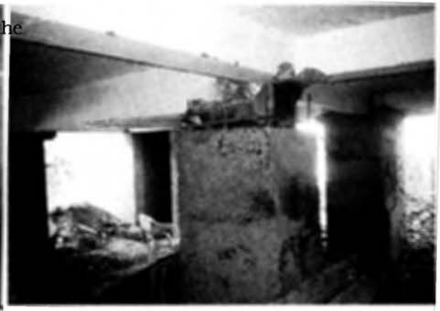
Photo 7.44 The connection between the reinforcement of the column of first story and the floor-beam of the second story was inadequate, leading to weak beam-column joint.
