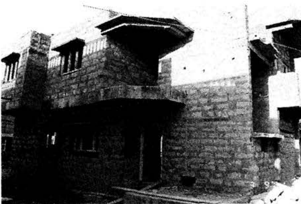
Photo 7.22 Huge stone masonry structure. Detail of a poor connection between RC beam and masonry wall, which might induce tension stresses on the wall
