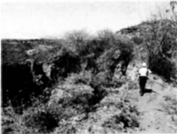
(a) Chang Dam
