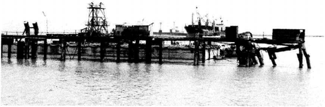
Photo 8.3. A view of damaged oil jetty at the Kandla port on March 19, 2001.
